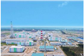
Rokkasho Reprocessing Plant
