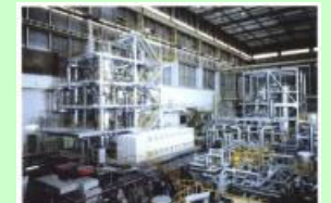
Helium Engineering Demonstration Loop (HENDEL)
